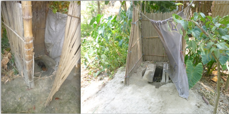
Figure 7: Left the 'hanging toilet' in Malbhanga, right the shared toilet without drainage in Malbhanga.
