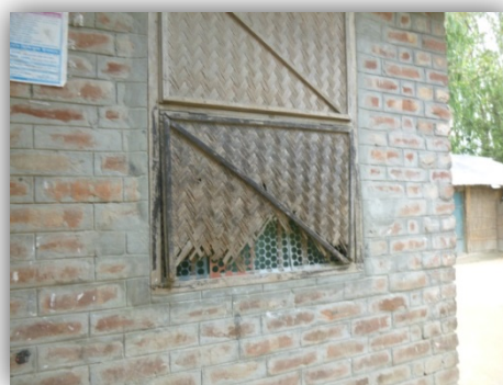
Figure 8: Repaired window in the Sreepur community.
