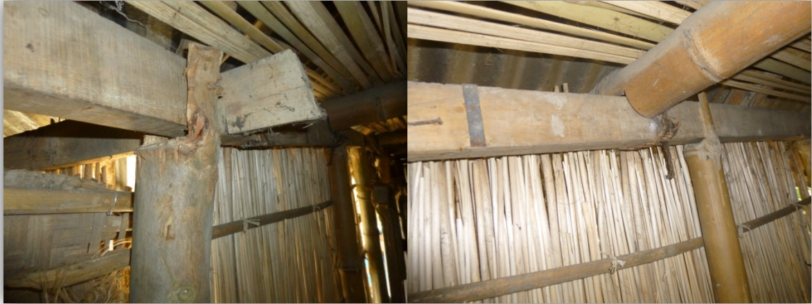
Figure 5: Provisionally repairs of wooden or bamboo made foundation in houses of the community Malbhanga.
