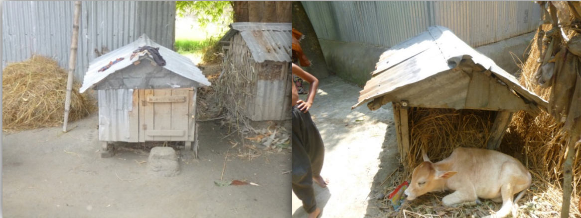
Figure 10: Little shed for chickens in the Malbhanga community. On the right the chicken shed is used for straw storage.
