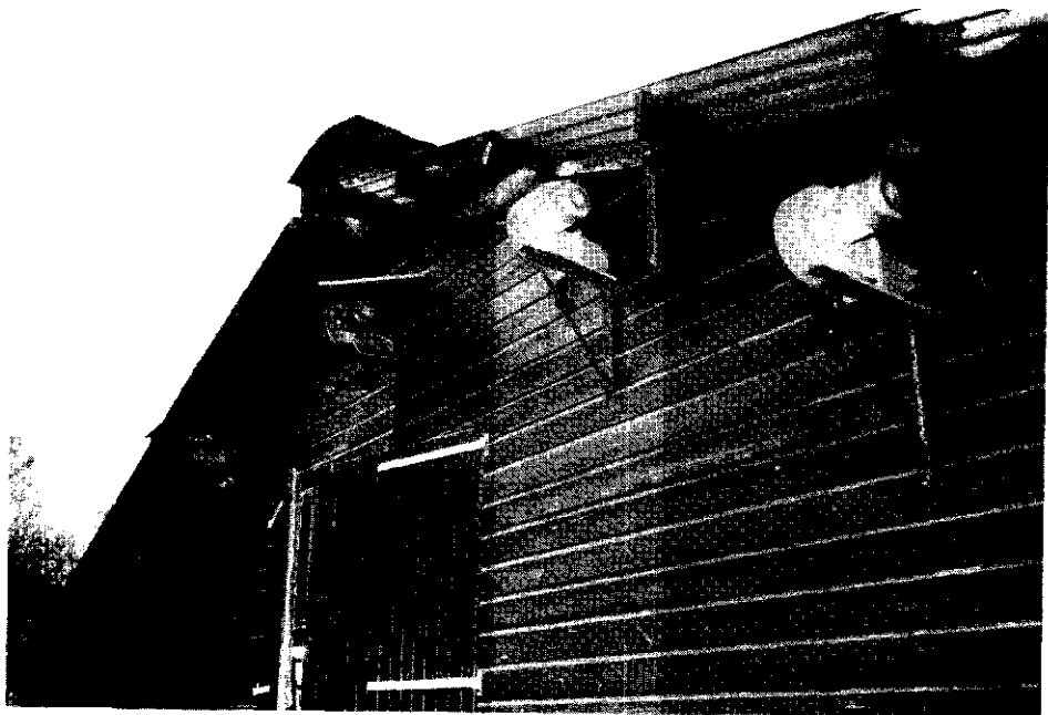
Fig. 3. In this stall a centrifugal fan has been connected to each battery
