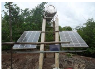
The salinity water treatment system using solar energy in Ca Mau Province
