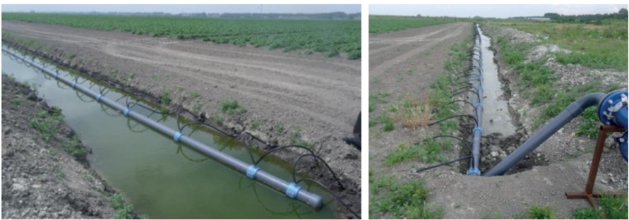
Figure 4: Subsurface irrigation using an innovative trickle system
