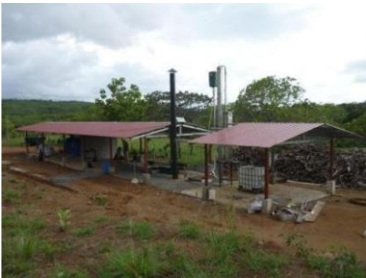
Figure 8. Small scale bioethanol plant designed for agricultural waste (e.g. cassava) installed in Panama (picture Agro2).
