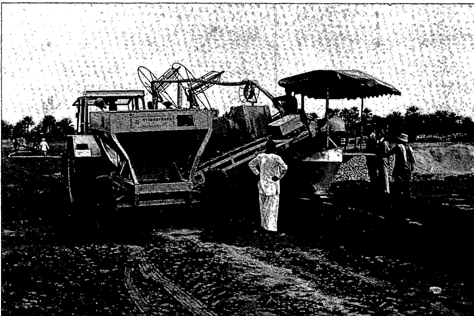
Figure 4 Self unloading gravel trailer for supplying into hopper of drainage machine, Pakistan
