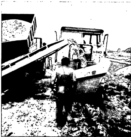
Figure 3 Installation of sand mole drains
