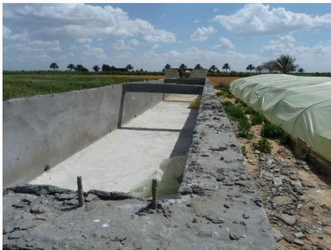
Left: new biofilter and fish basin (under plastic) under construction. Right: small back-yard recirculation system with trickling filter tower at the rear and fish basin in front.
