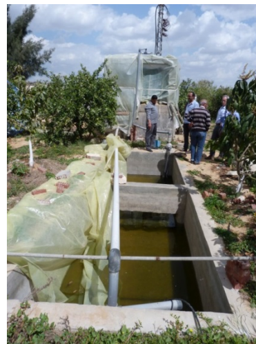
Left: new biofilter and fish basin (under plastic) under construction. Right: small back-yard recirculation system with trickling filter tower at the rear and fish basin in front.
