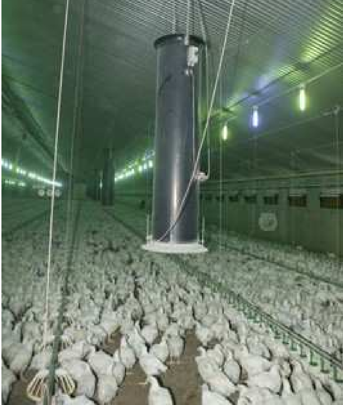
Figure 2. Photograph of the experimental broiler house with an air circulation unit in the front.
