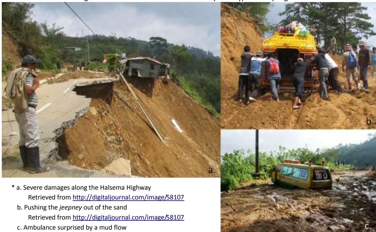
Figure 7.1: Bad road conditions near Tublay after typhoon Pepeng*
