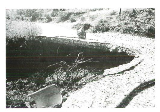
Fig. 2.5 Road near profile Sp/234, destroyed through vertic processes under the road surface and insufficient drainage measures. Note crack at the left side of the picture, extending to the surface and breaking up the road.
