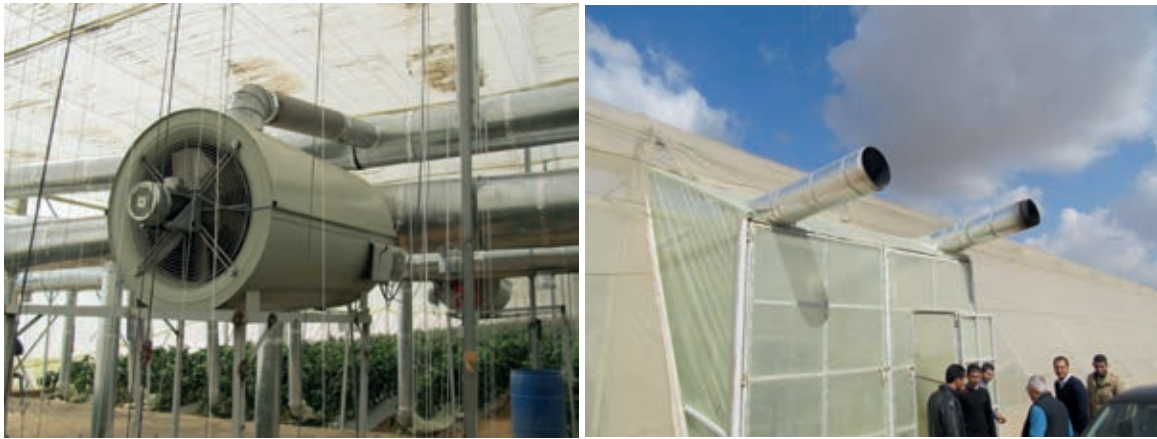
Figure 6. The diesel operated heating system at AllGreen (left) with exhaust pipes to the outside (right).
