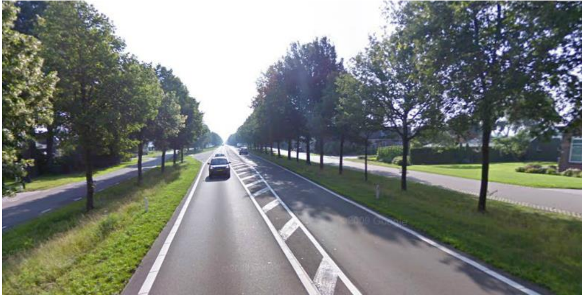
Figure 40: Parallel roads to separate the slow and fast motorized traffic (source: Google Street view)
