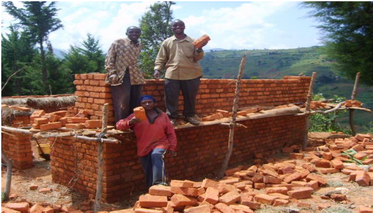
Photo 6.3: Author with 2 masons constructing classroom walls in Bwishasha primary school, Burhinyi
