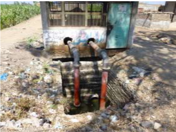
Figure 26 - Newly constructed pit for water collection (23-06-2013)
