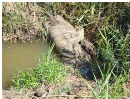
Figure 35 - Farmers have blocked the north Hosha drain in PS31 (26-07-2013) (See also: Figure 38)
