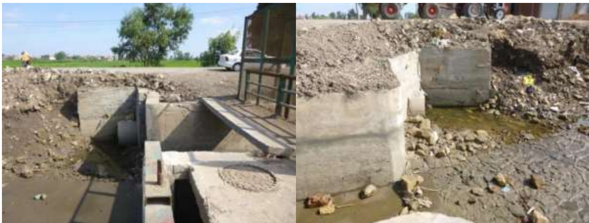
Figure 10 - Newly constructed pipeline past the AVIS gate in Abo Moustafa canal (3/8/2013)
