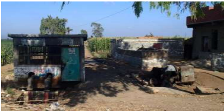
Figure 23 - From left to right: PS33, individually owned pumps, unused valve (28-06-2013)
