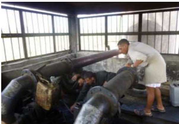
Figure 28 - The operator and treasurer discussing with the mechanic about the problem
