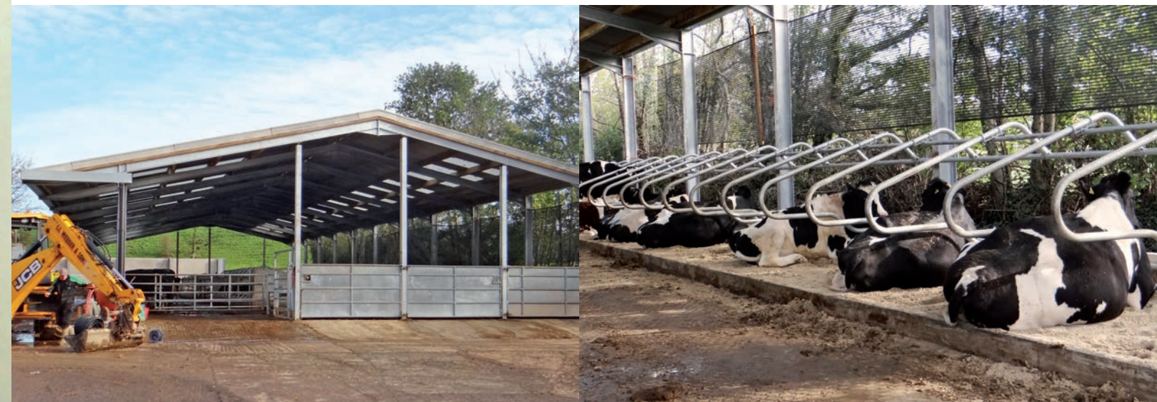
New shed: improved cow housing, with sand-bedded cubicles, has played a key role in reducing the incidence of mastitis
