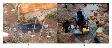
Figure 9.3: A) Grey water from a bathroom stagnant beneath a water meter for a piped water supply house connection in Bwaise III and B) Evidence of exposure to contaminated and unprotected drinking water in Bwaise III
