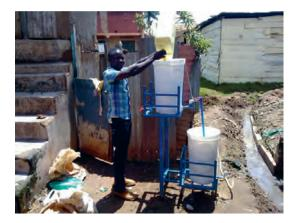
Figure 9.5: A crushed lava rock filter for grey water treatment by a household in Bwaise III
