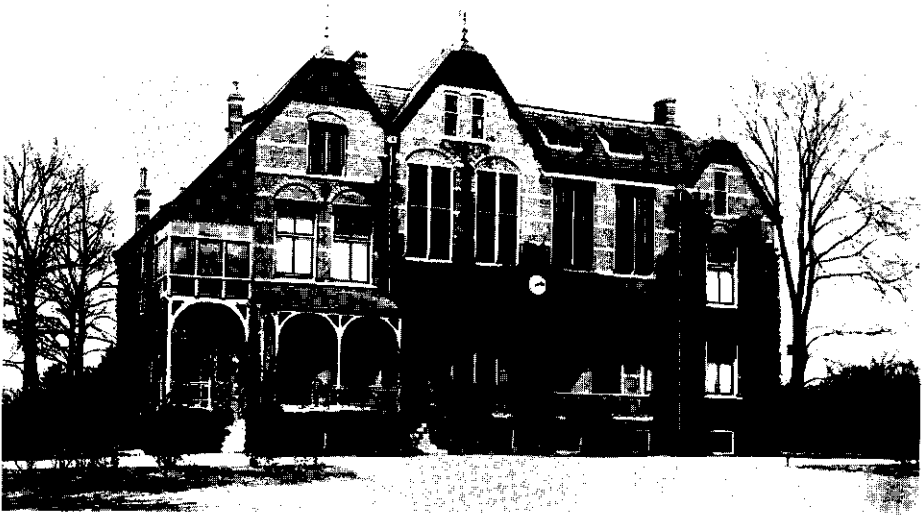
Fig. 1. The building of the State Horticultural College in early 1900; later on the Department of Plant Taxonomy was housed in this building.
