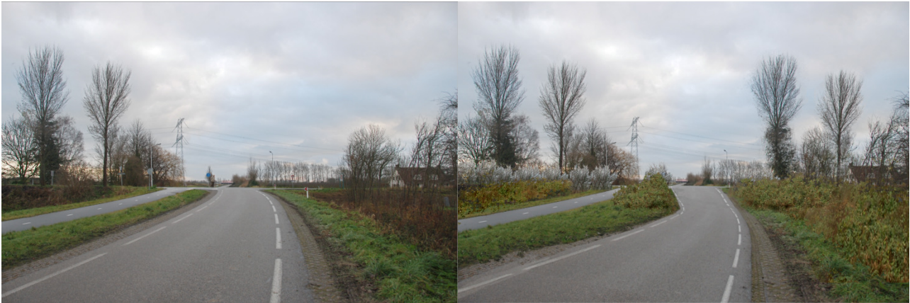
Fig. 7. Dangerous connection of a road not situated on a dike with a dike road (on the background). Left: in the present situation the road in front leads fluently to the dike road, making the dike invisible. Right: the proposed solution is to accentuate the characteristics of the dike road by planting trees on the dike and a less fluently bend with a sharper slope of the other road (Van Blerck et al., 2009).
