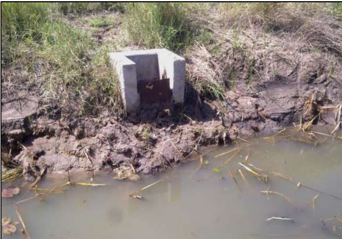
Figure 7: Tertiary canal intake in which is possible to see the results of the rehabilitation which lowered the secondary canals, consequently it is necessary more water to reach the intake.
