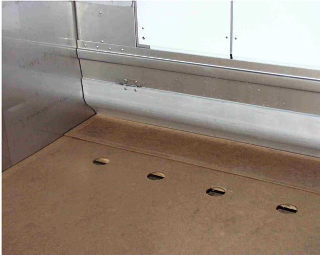
**Fig. 7, chink at unit end closed with board.**
