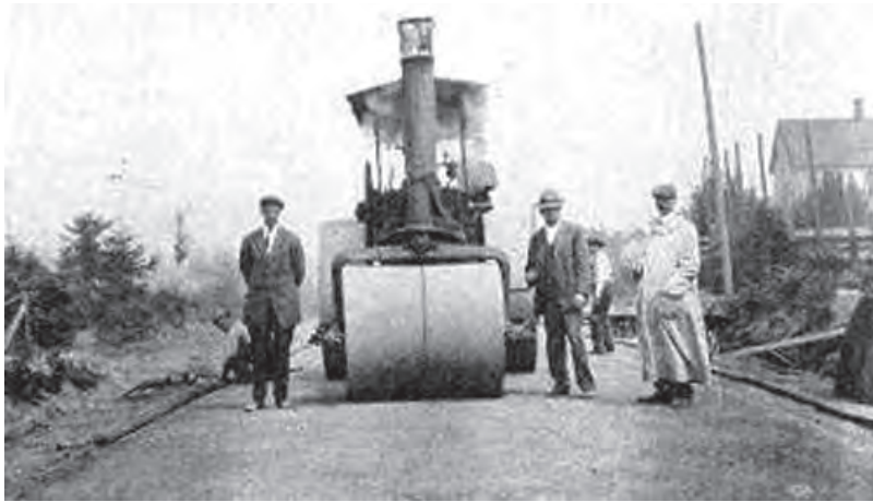
Steam powered roller on asphalt pavement, 1934
