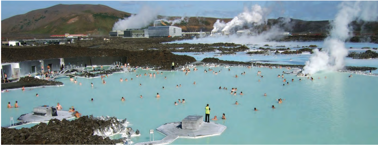
Post-Carbon Resource Park: view of the Svartsengi Geothermal Power Station in southwestern Iceland where geothermal effluents are re-circulated through a public health spa and wastewater lagoon, rich in blue-green algae, mineral salts and fine silica muds. Source: ©2009 Stephen Bunch
