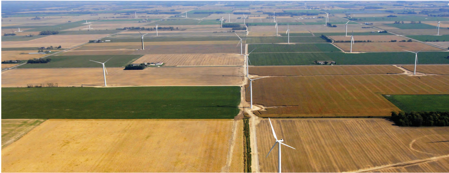
Farmland & Power The first commercial scale public utility wind field in Michigan built by John Deere Renewables on land leased from cooperative sugar beet farmers near Bad Axe. Source: Don Coles, Great Lakes Aerial Photography, 2008.
