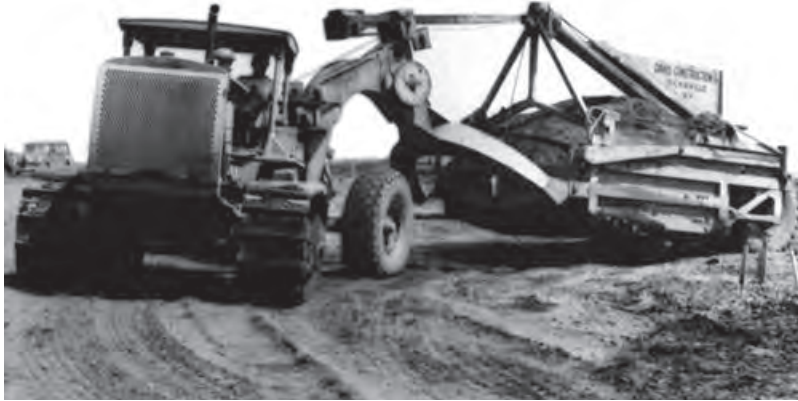
The revolutionary tournapull, 1948. The first integral, articulated wheel tractor scraper earthmover, developed by Robert G. Letourneau
