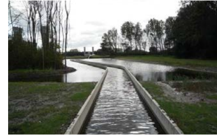
Figure 6.25 Flowing water retention along an urban stream source: http://www.bplusb.nl/?project=wijkeroogpark-velsen
