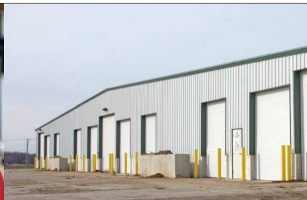
New building: the cross ventilation barn
