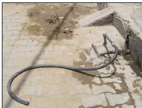
Picture 4.2: Plastic pipe used for connecting to water supply
