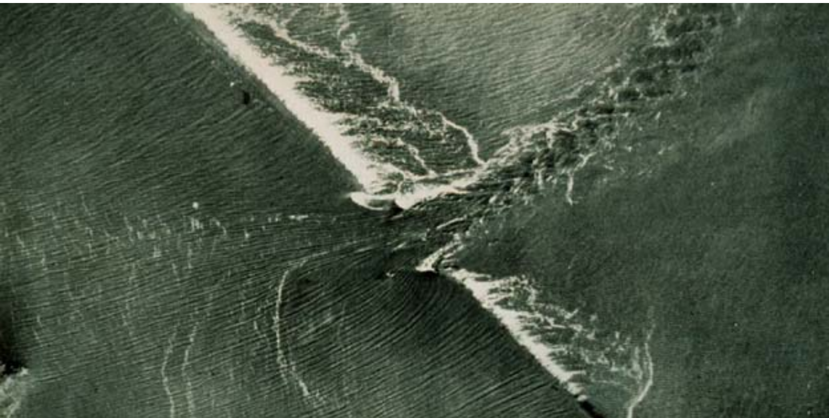
Figure 2.6 | 1927 Mississippi Flood Levee Breach (source: commons.wikimedia.org).
