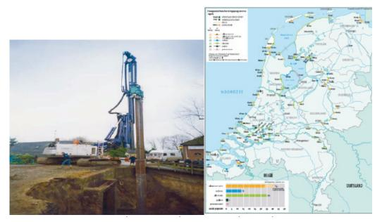
Figure 44: Repairing a drainage culvert using sheet piling Figure 45: HWBP measures
