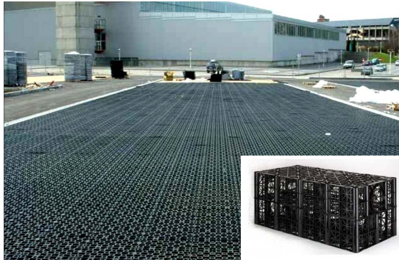
Figure A.3.9 Geocellular System Image (CIRIA, 2007, p38 )
