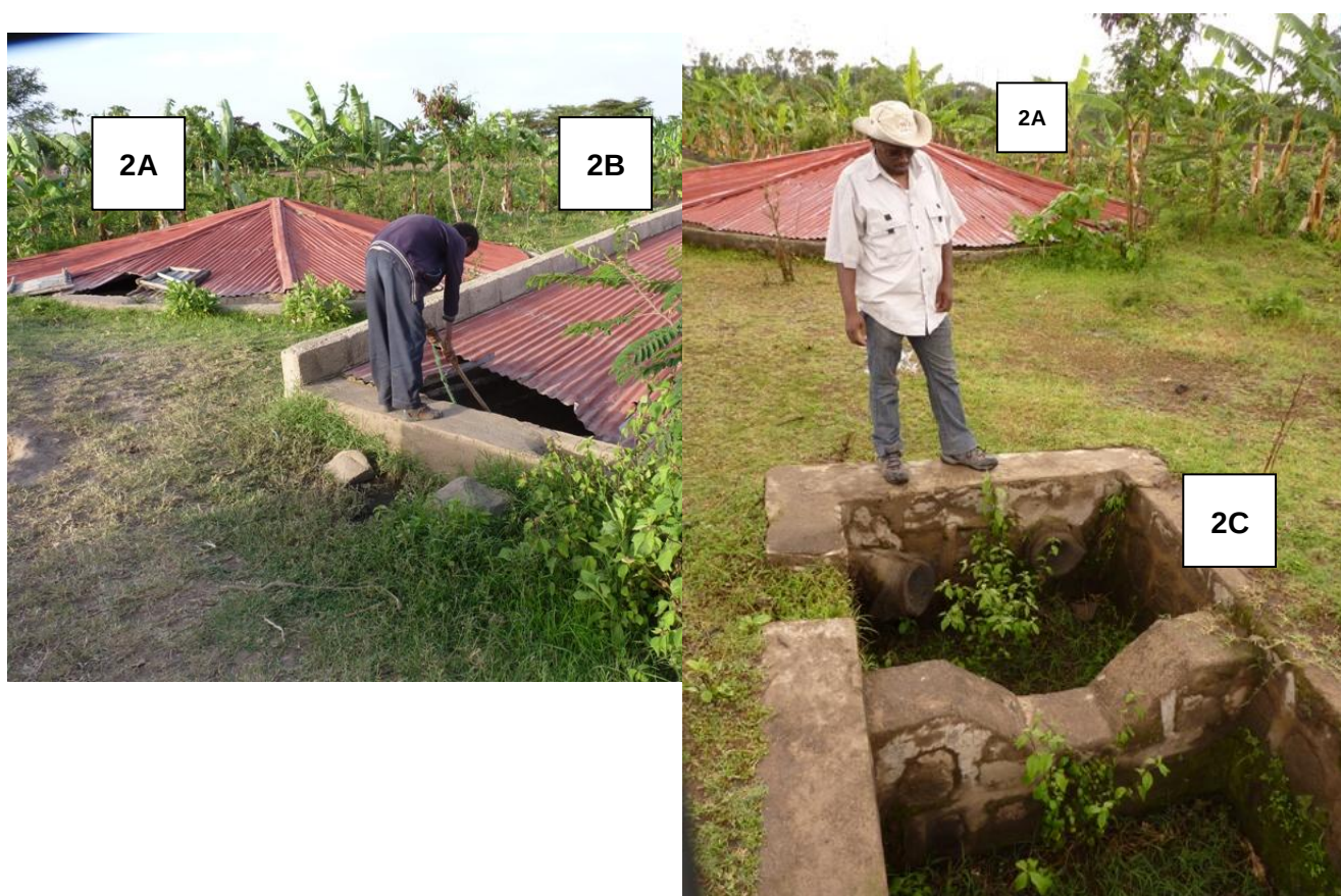
Figure 7 Pictures of the two Rainwater Harvesting cisterns (1 and 2), each with a round basin (A), a square basin (B) and a silt trap (C).
