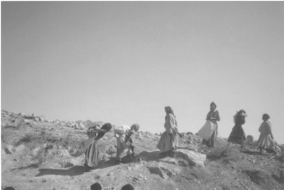
Photo 7.1 Women carrying bags of soil at Shelenat dam construction site
