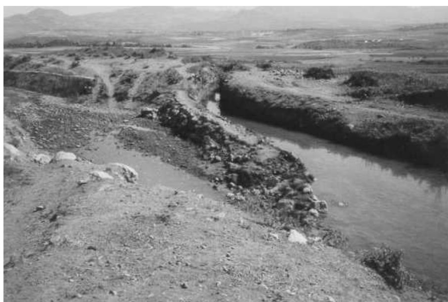
Photo 3.1 An outlet constructed by hayfo irrigators cutting Shelenat diversion canal at Korkora
