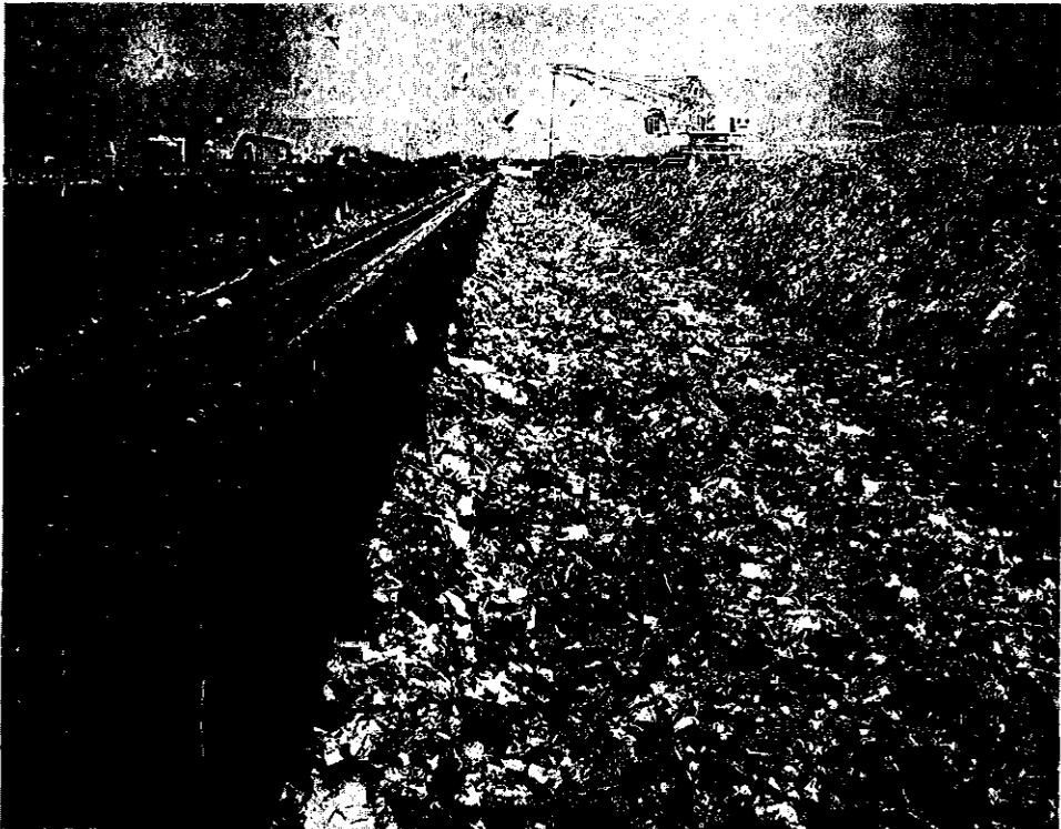
Fig. 1. One of the four railway tracks along which the refuse is transported, and the adjoining refuse windrow, at the compost plant of the VAM Waste Disposal Company at Wijster.
