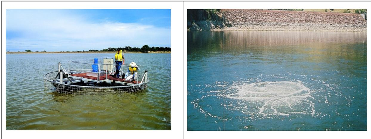
Figure 4-2 Mechanical mixer (left) and aerator (right) at Myponga Reservoir
