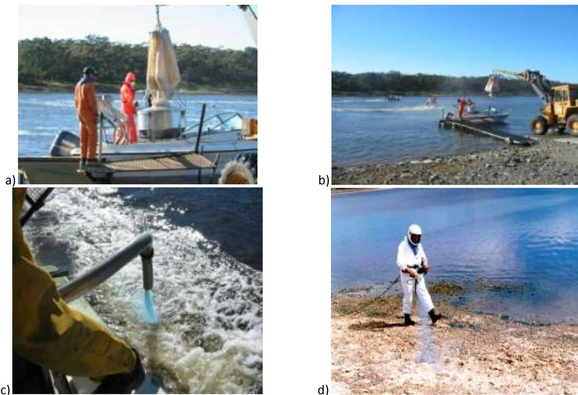
Figure 4-5 Copper sulphate dosing of a reservoir (a-c) and benthic cyanobacteria after reservoir draw-down d)
