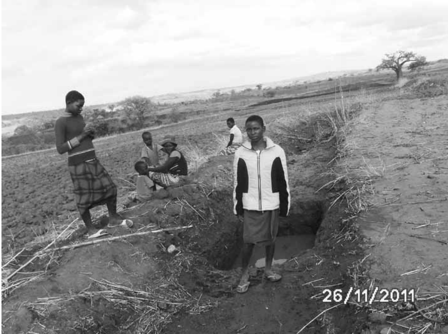
Figure 2 Example of local water conservation: infiltration pits in channels upstream of conservation ridges in Zimbabwe (Photo by Innocent Nyakudya)
