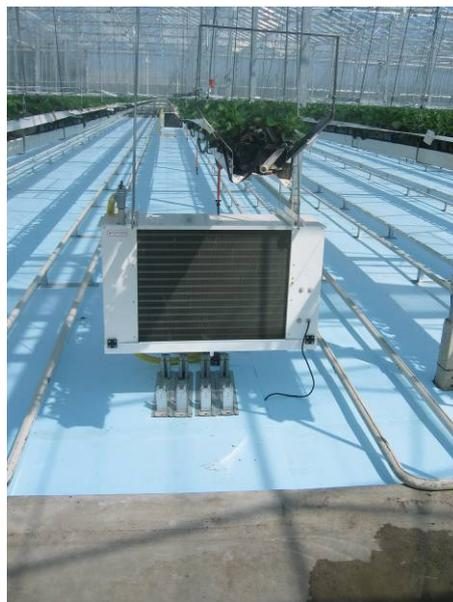
Fig. 2. Cooler in section 3 with insulation plates.
