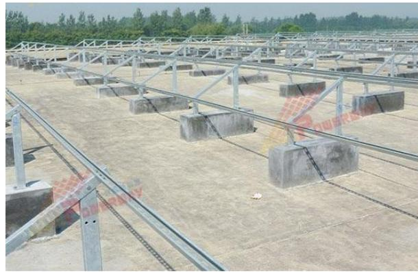
Figure 26 Multiple rows of PV frames on concrete foundation and at regular spacing ([www.pvpowerway.com/news/769.html](http://www.pvpowerway.com/news/769.html))
