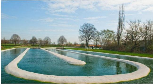
Figure 14 Open raceway pond (Wolkers et al., 2011)
