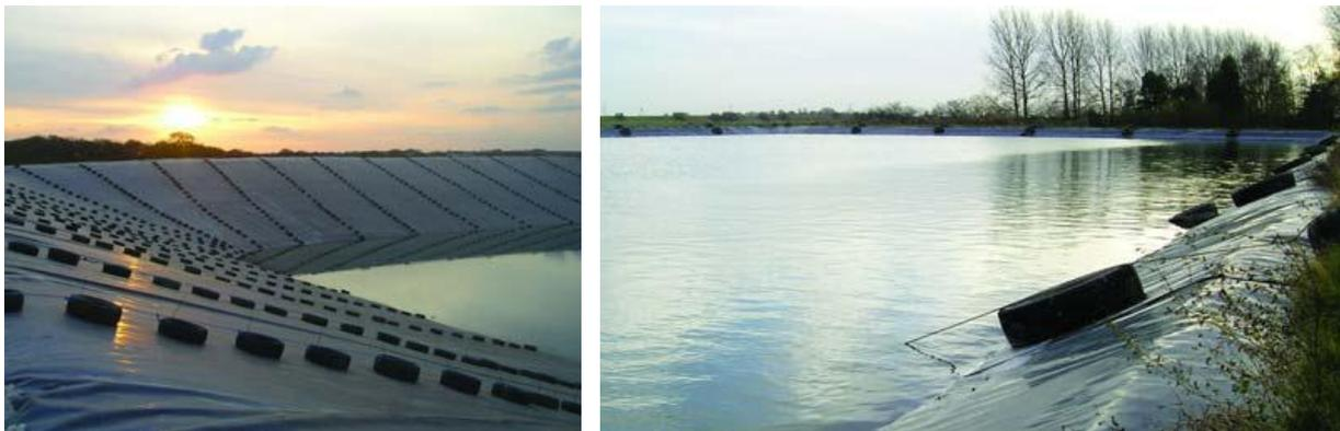
Figure 22 Pictures of a lined basin (adapted from Weatherhead *et al.*, 2008)
