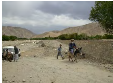
Flood wall along dry riverbed
