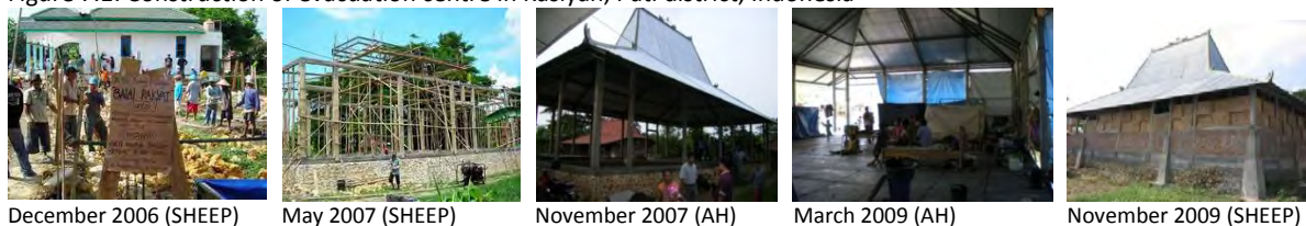
Figure 7.1: Construction of evacuation centre in Kasiyan, Pati district, Indonesia
