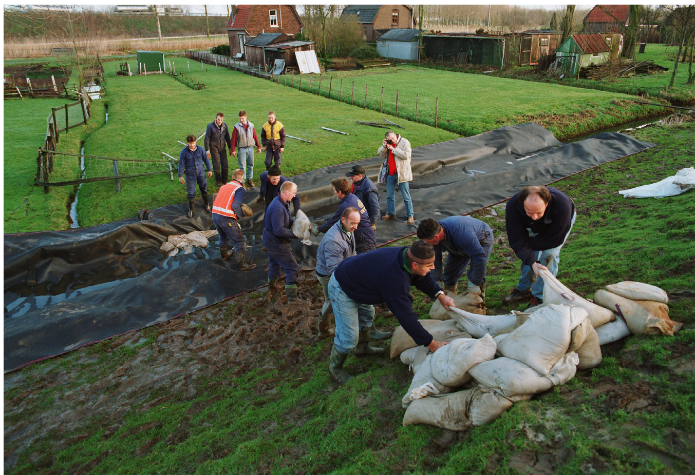
Photo 2. Stopping seepage through a Dutch dike with sand bags
