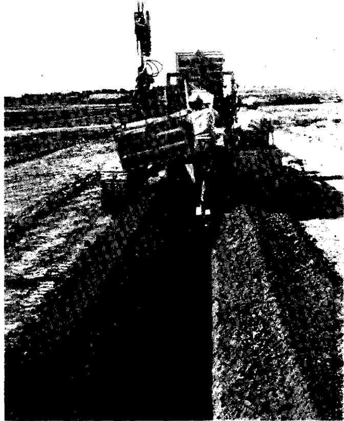
*Fig.7.7: Installation of clay drains.*
