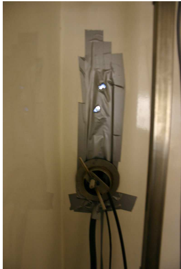
Fig. 3, holes drilled into vent opening (inside view).
