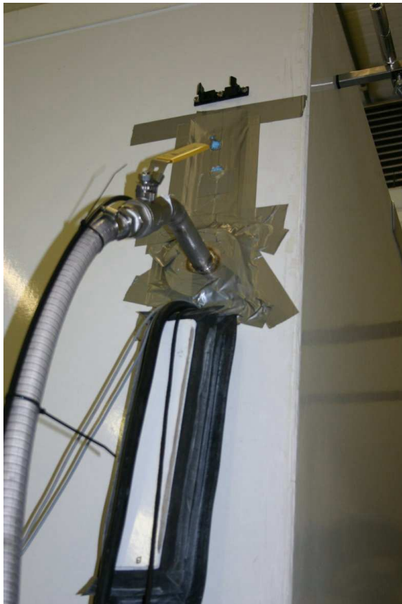
Fig. 2, holes drilled into vent opening (outside view).
