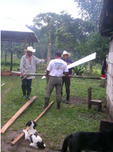
Pic.6.28 Juan, Pedro and Jerónimo building the roof
