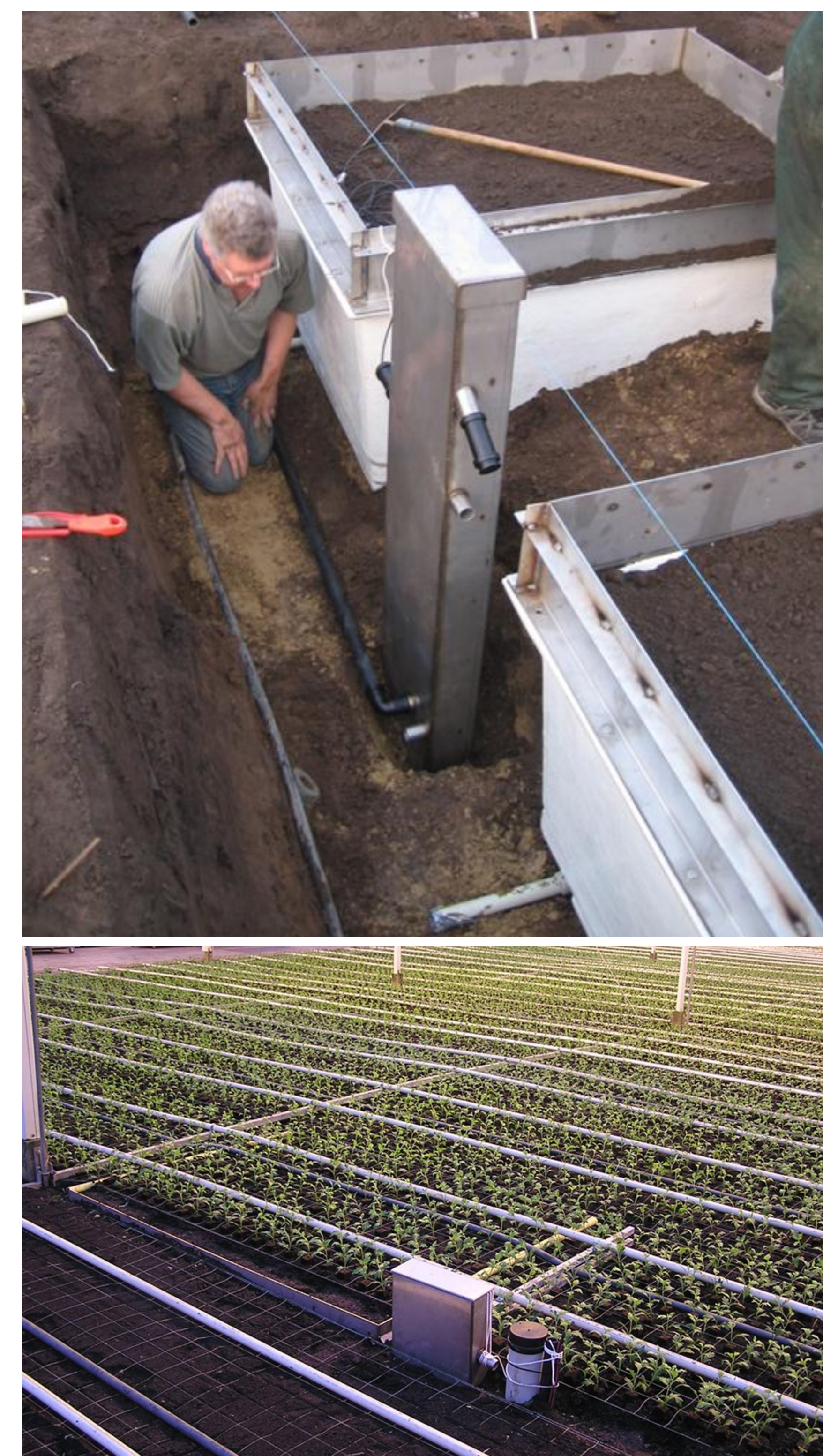
Figure 2. (top) Installation of the lysimeters, and (bottom) top view after installation.
