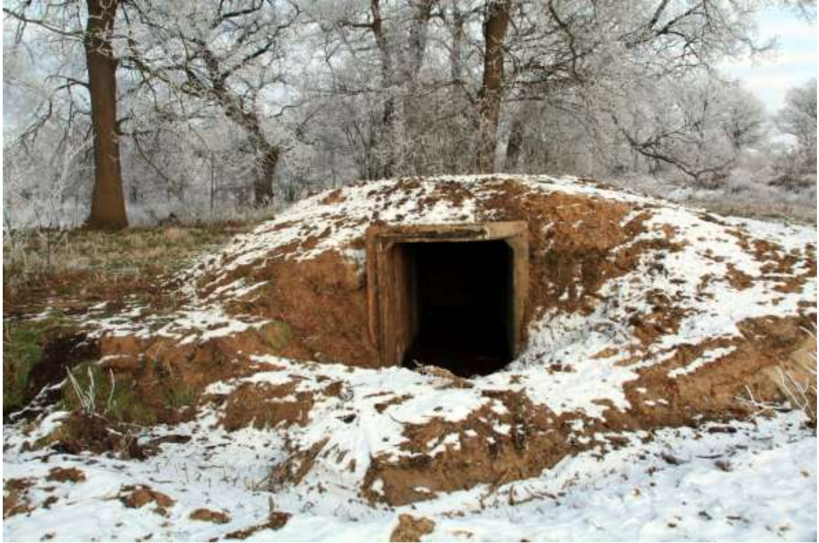
Figure 37: The new bat habitat
