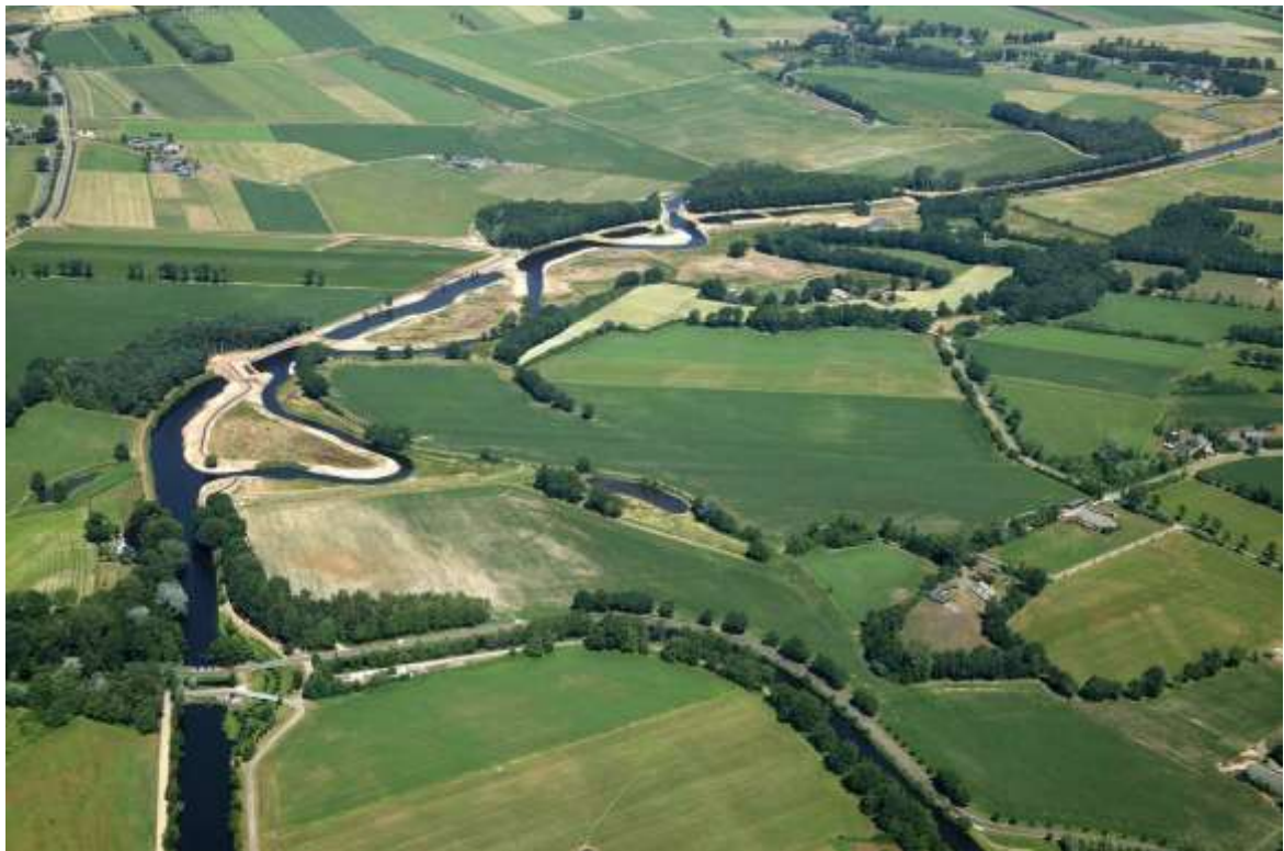
Figure 46: Aerial picture of Velderberg area
