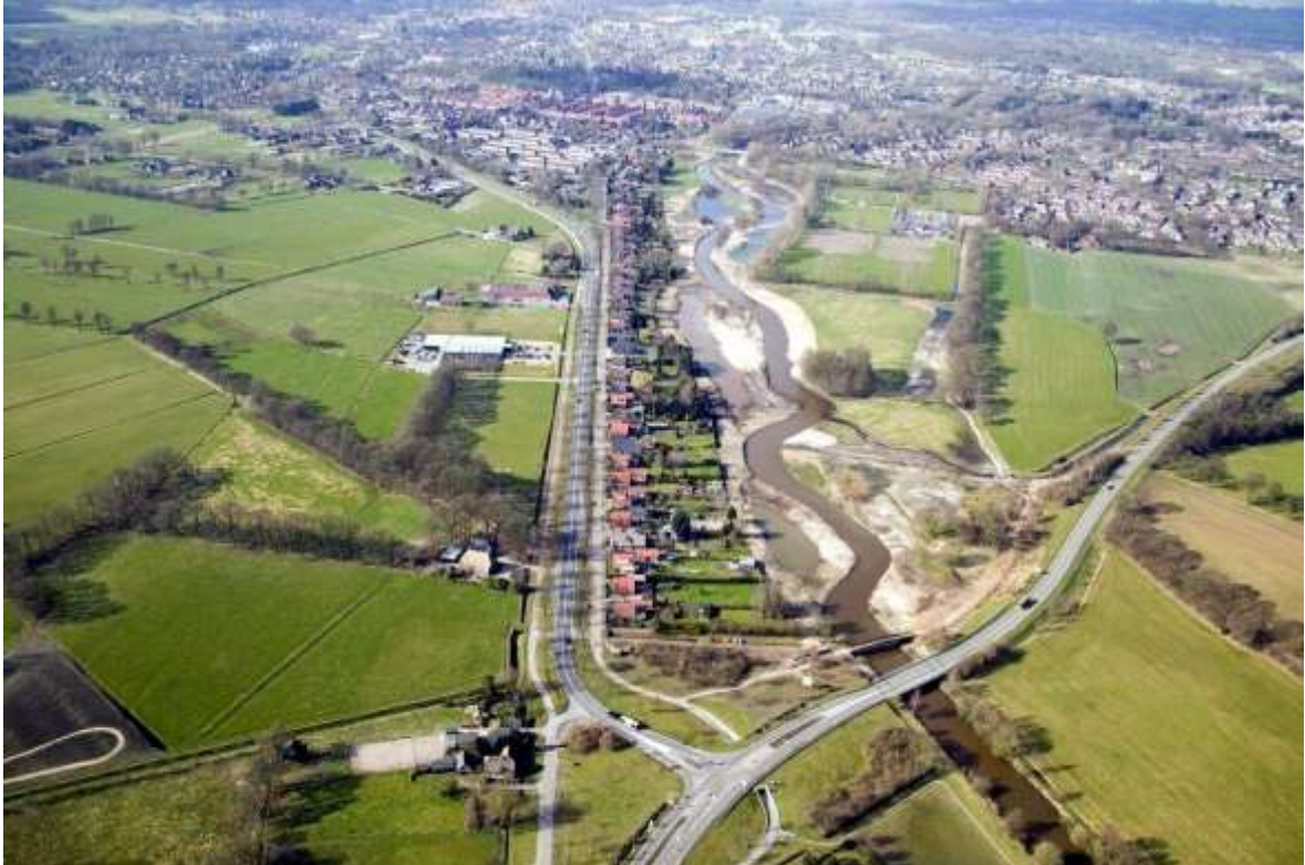
Figure 39: Veldkamp work in progress (Source: Photo Holland)
