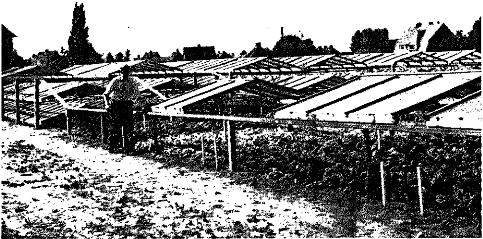
FIG. 10. The application of glass shelters from the depot
