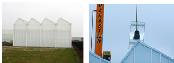
FIGURE 1. Impression of the 480 m 2 Fresnel greenhouse with 4 roof spans with Fresnel lenses mounted at the south facing roof segments.
