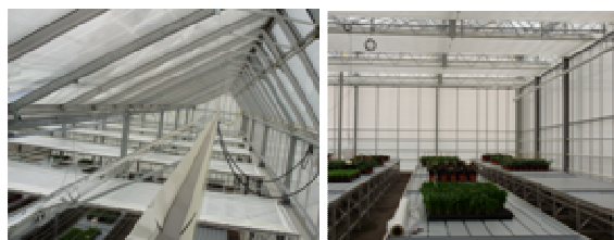
FIGURE 4. Left: Details of the receivers inside the greenhouse with two receivers per roof. Right: the cultivation area with pot plants in the greenhouse (still only half filled).
