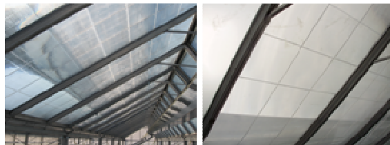
FIGURE 2. Details of the modular constructed Fresnellens. Each lens is assembled from 12 parts and two lenses are mounted in one double glass pane.
