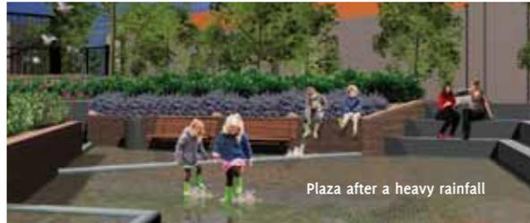
**Bellamyplein, Rotterdam, NL** | Bellamyplein, a multifunctional water plaza designed by ds + v, afdeling Stedenbouw, has the capacity to hold 750 m<sup>3</sup> water during extreme rain in order to ease the storm sewer system in the neighbourhood of Spangen. The plaza is 90% of the time dry | Photo: Gemeente Rotterdam, afdeling Stadsontwikkeling
