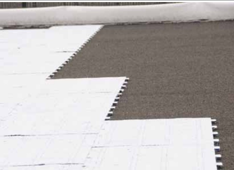
10 Installatie shockpad Schmitz Foam.
