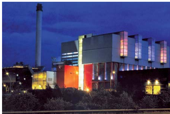
Tyseley Waste-to-Energy plant, Birmingham, UK. Built in 1996, the 28 MW plant with a 2-stream incinerator has a combined capacity of over 350,000 tonnes per year of municipal solid waste and a fifteen year Non-Fossil Fuel Obligation Contract. An award winning lighting system illuminates the plant at night.
