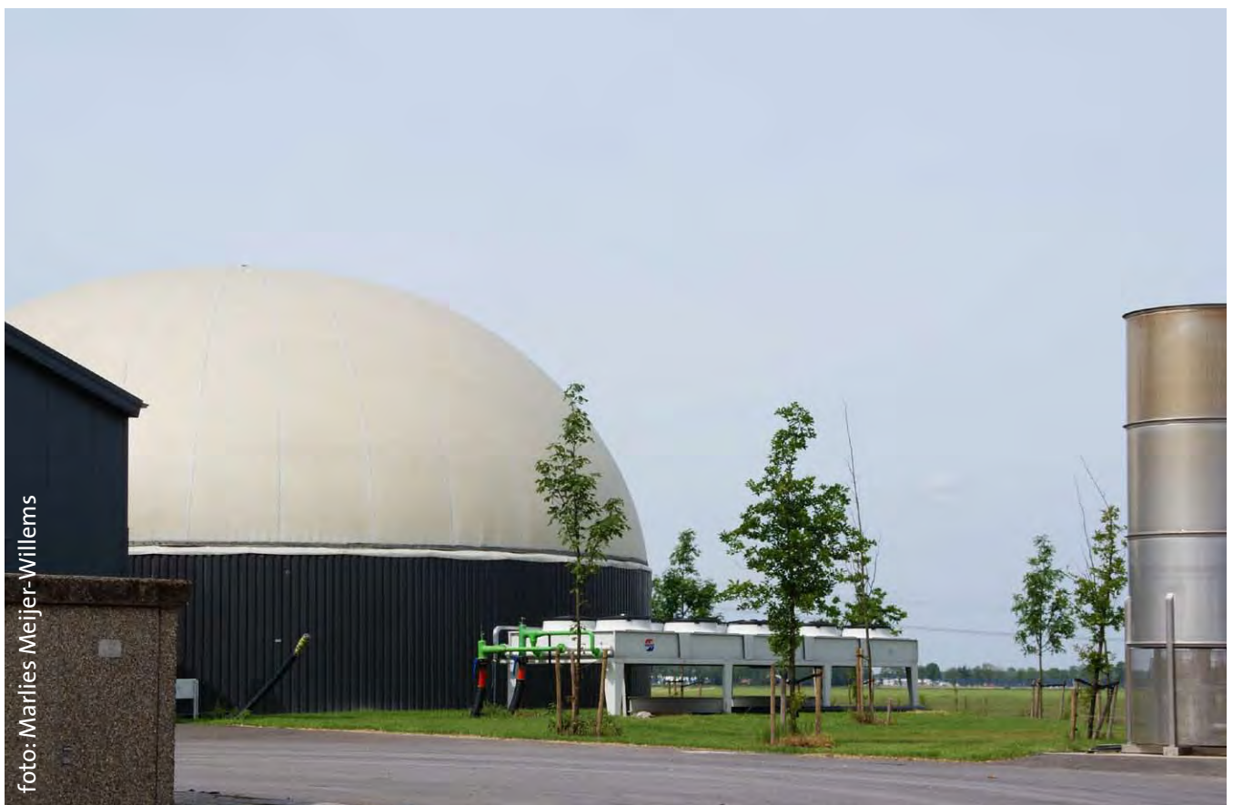
Figure 4.2 Biodigester at the Steegro dairy farm
