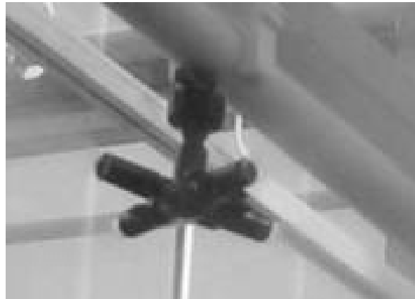
Fig. 3. A four headed nozzle of the mist system during misting.
