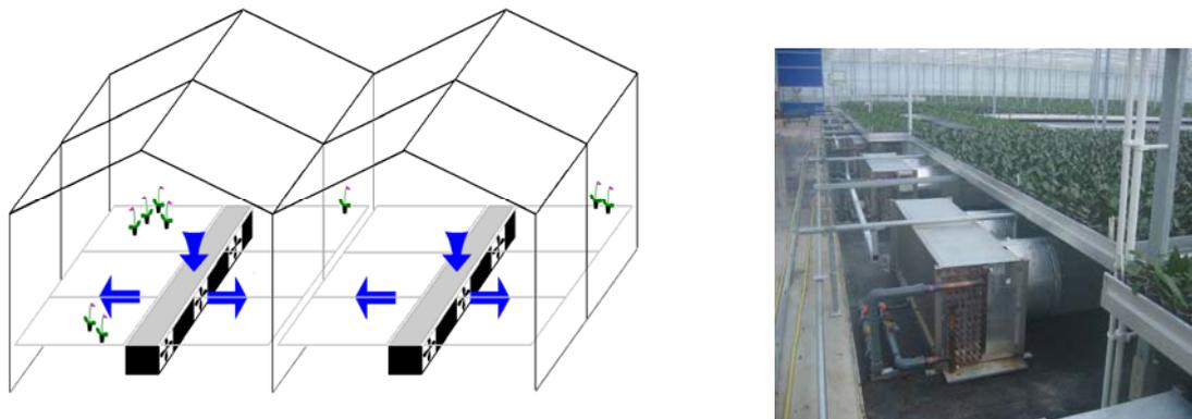
Fig. 2. Moving benches with pot plants (*Phalaenopsis*) and the air conditioning system consisting of decentral ACBs (left) and central ACBs with perforated air ducts (right).
