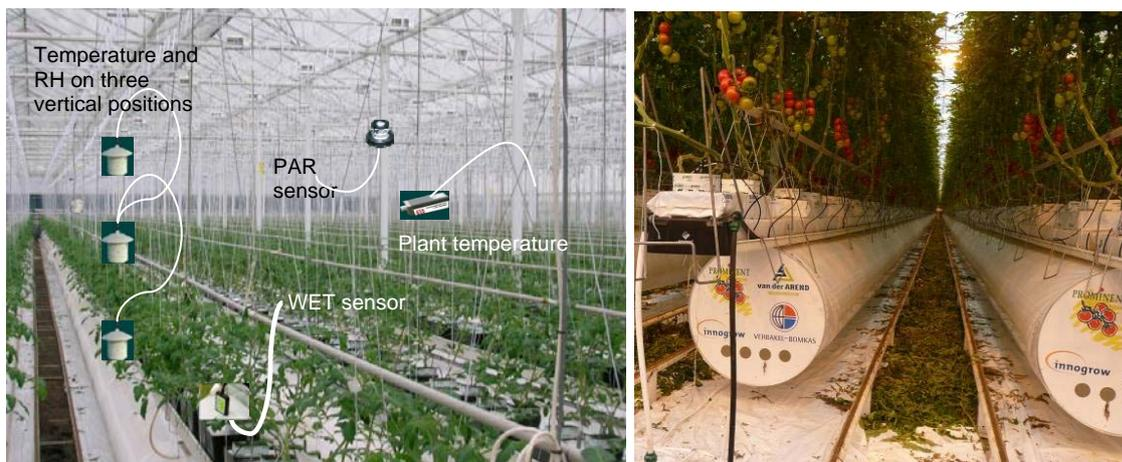
Fig. 1. Sensors situated in a greenhouse with a tomato crop (left) and air ducts of a decentralized system below the crop (right).
