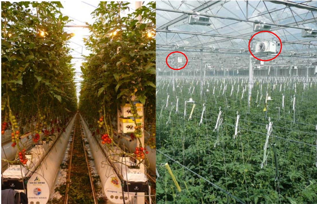
Fig. 1. Picture of a greenhouse with air ducts positioned beneath the hanging gutters (left) and a picture of a greenhouse where the coolers are hanging above the crop near the cover of the greenhouse (right).
